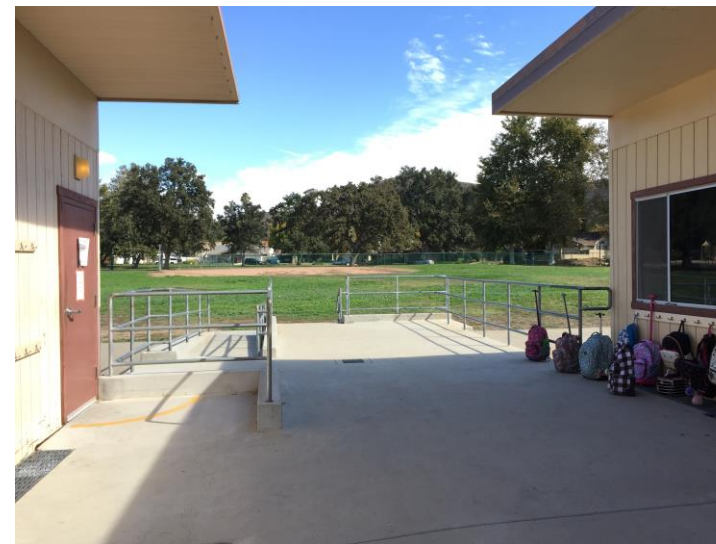
Photo 3 Image showing recent improvements to accessible path of travel.
