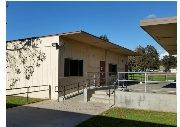
Photo 2 Image showing recent improvements to accessible path of travel.
