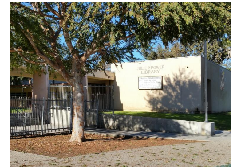
Photo 4 Image showing recent improvements to accessible path of travel.
